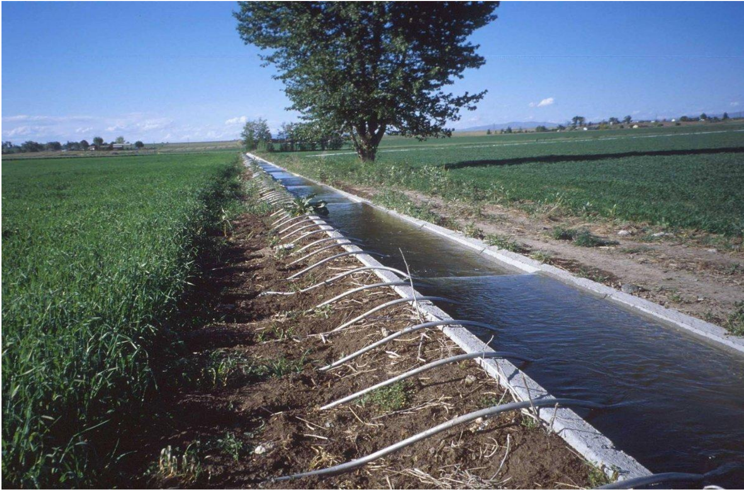
Fig.1: It shows open channel flow as well as pipe flow (Syphon) for irrigation
