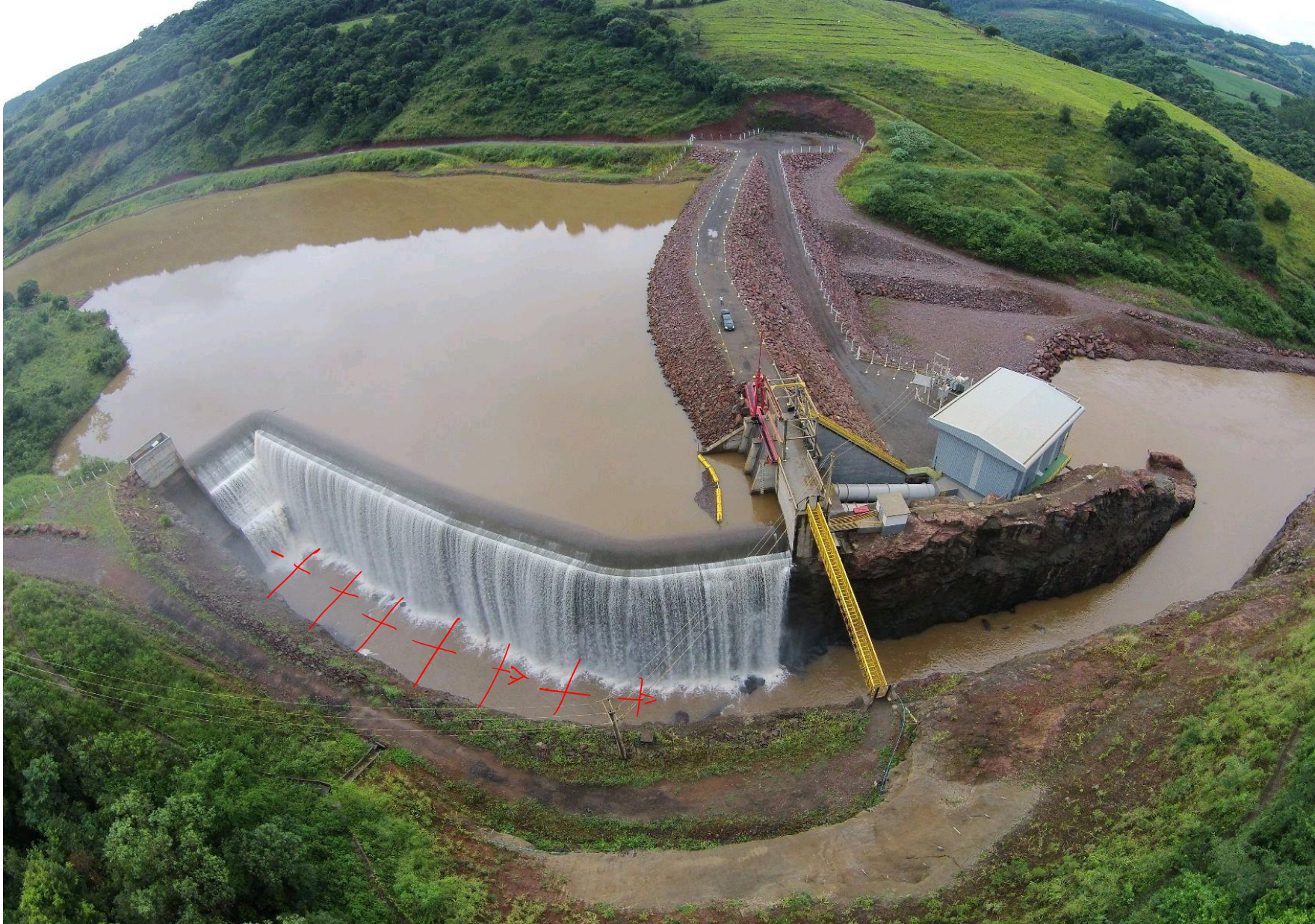
Fig: Side-channel spillway as an example for spatially varied flow
